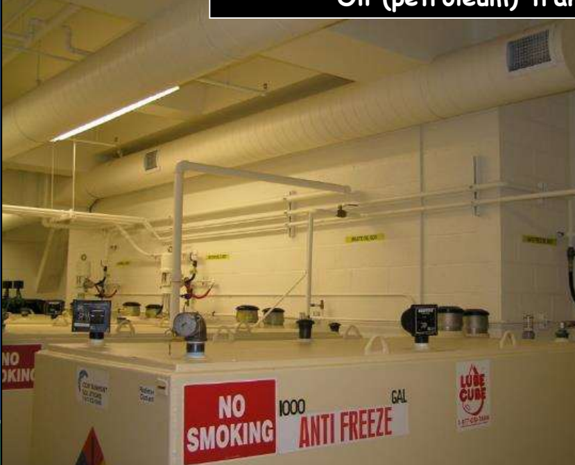
Oil (petroleum) transfer areas (piping)
