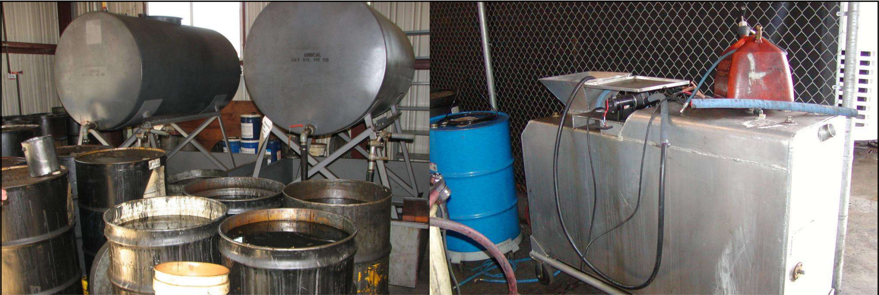
Bulk storage containers (stationary ASTs) & portable bulk containers (drums)
