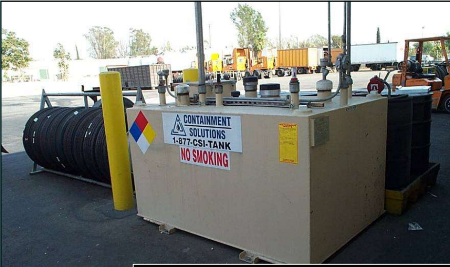
Bulk storage containers (stationary ASTs)
