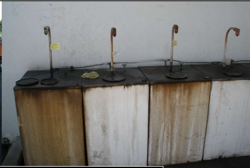
Bulk storage containers (stationary ASTs)
