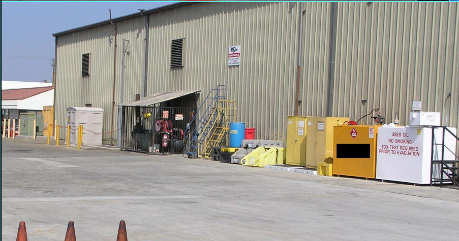
Bulk storage containers (stationary ASTs) & portable bulk containers (drums)... and oil transfer area
