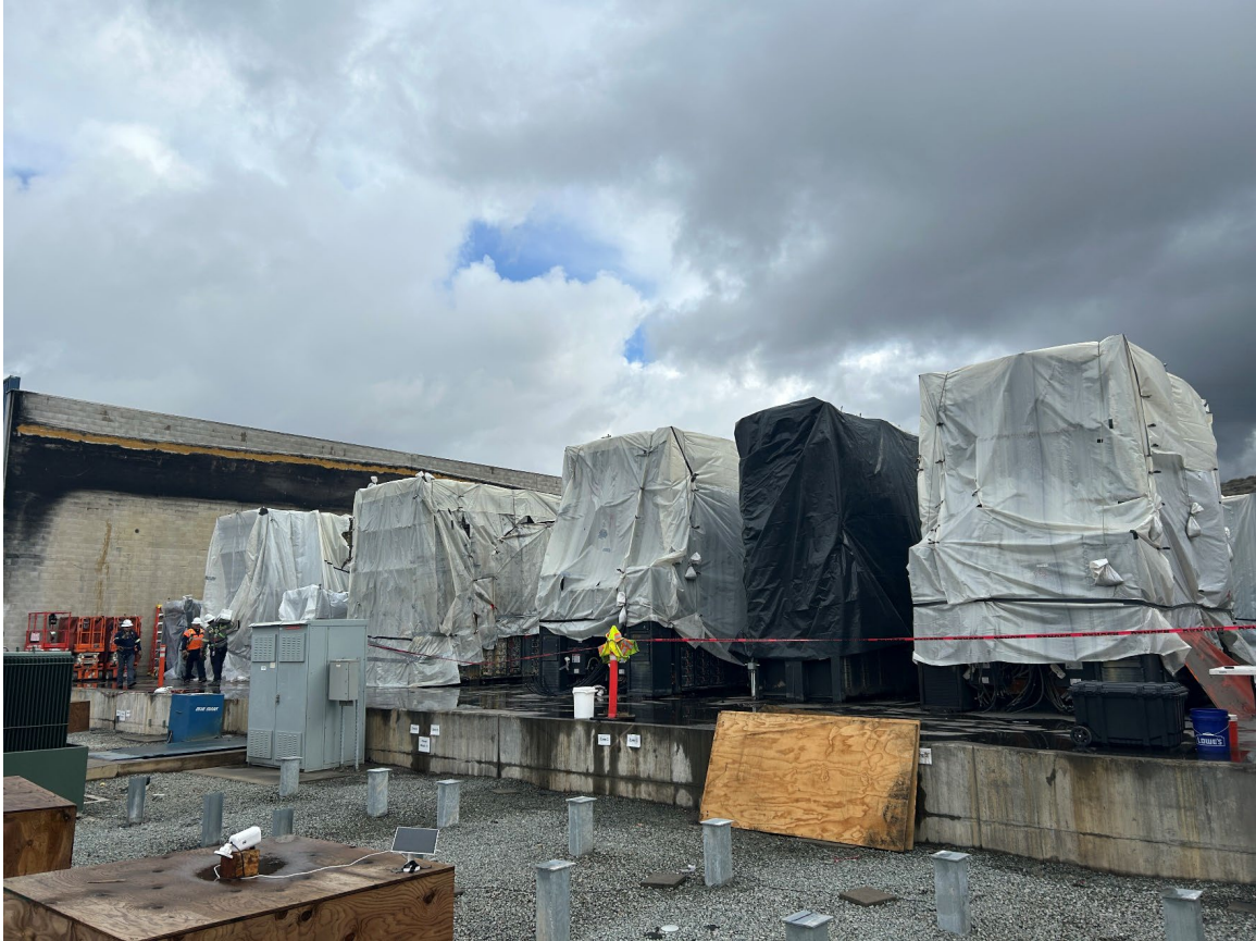
Roof removed, Battery racks wrapped to prevent rain impacts
