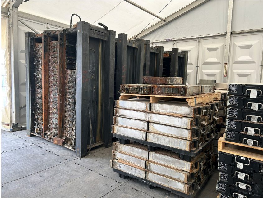
Staging, Assess voltages, remove battery cases
