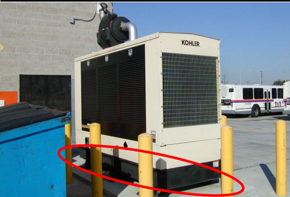
Bulk storage container (stationary AST)
