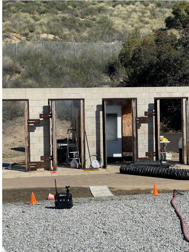
Photograph F: Note the heavy amount of off-gassing matter through the shed door window and the off-gassing on the left side of the shed walls. An AreaRAE monitor provided by SDFD monitors for gaseous migration at the perimeter of the Hot Zone.
