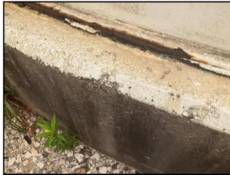
003 Spalling on Ringwall
