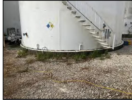
002 Grade Surrounding Tank Foundation
