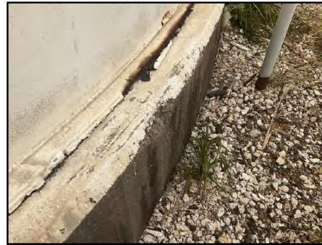
004 Spalling on Ringwall
