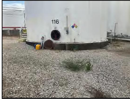
001 Grade Surrounding Tank Foundation
