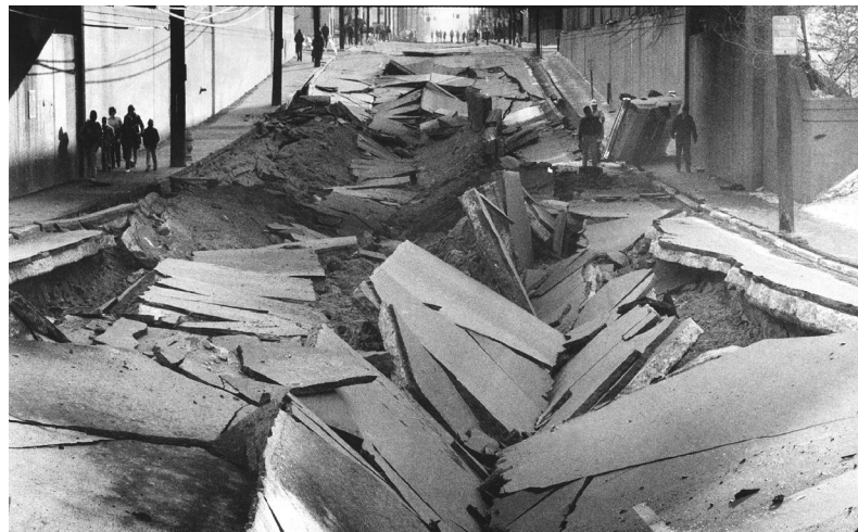
1981 Louisville Sewer Explosion
