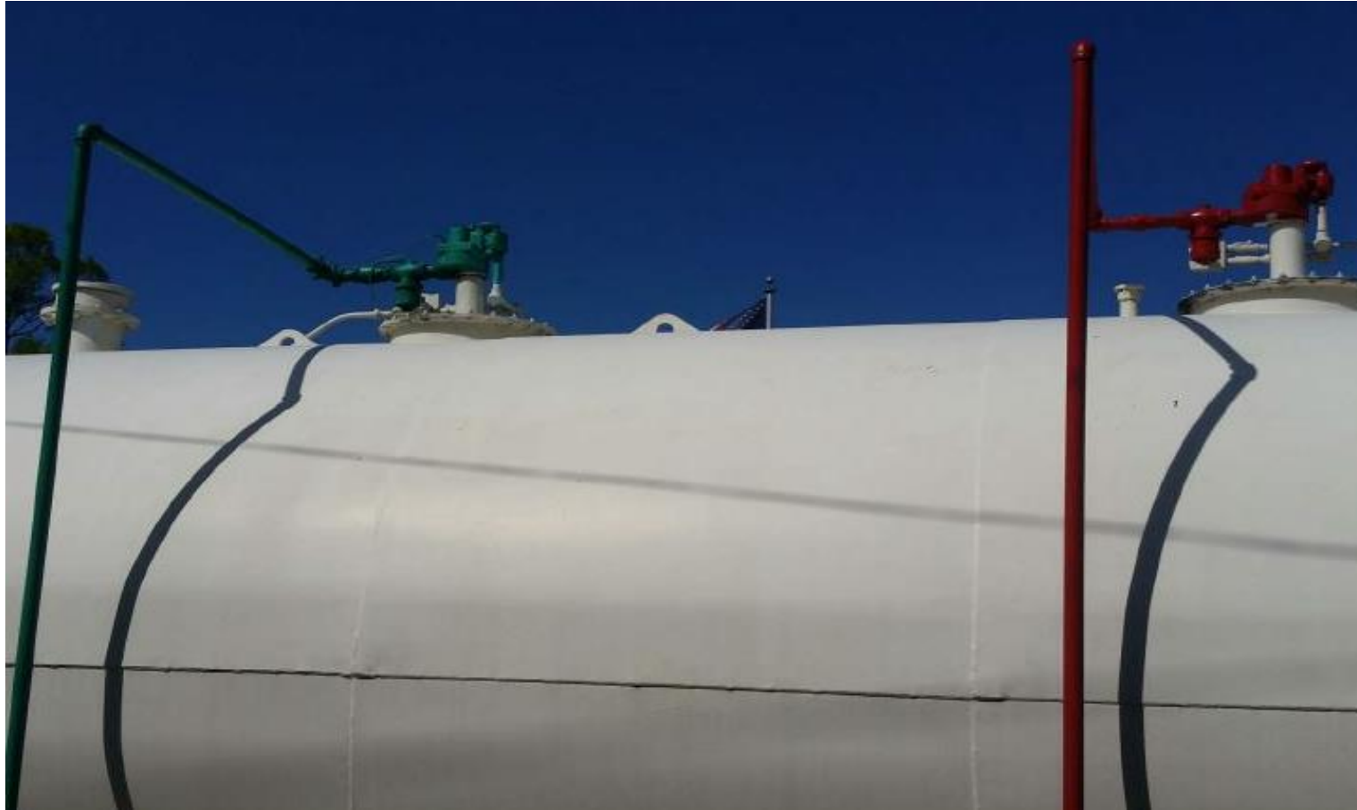
Anti-Siphon Valves installed upside down
