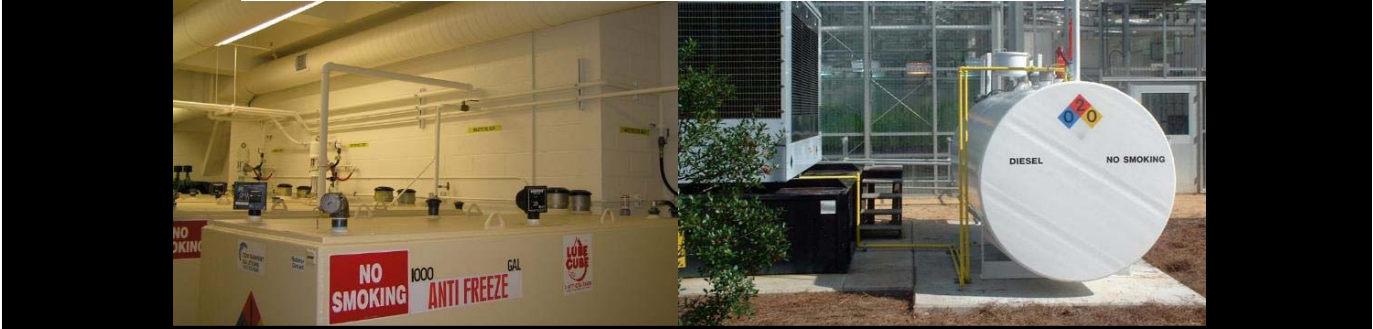
Oil (petroleum) transfer areas (piping) Containment for most likely/typical failure (general containment) reqd.
