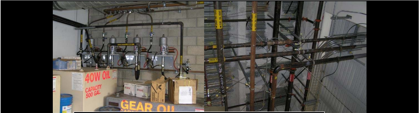
Oil (petroleum) transfer areas (piping) Containment for most likely/typical failure (general containment) reqd.
