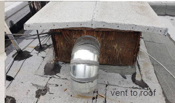
new ceiling vent and exhaust
