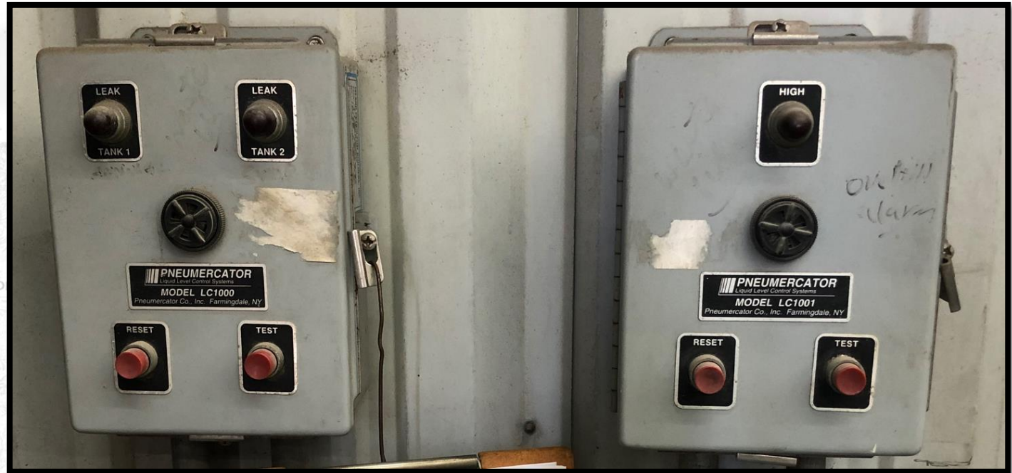
LC 1000 and 1001 (Hi Level Panel)
