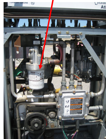
Filter inside dispenser
