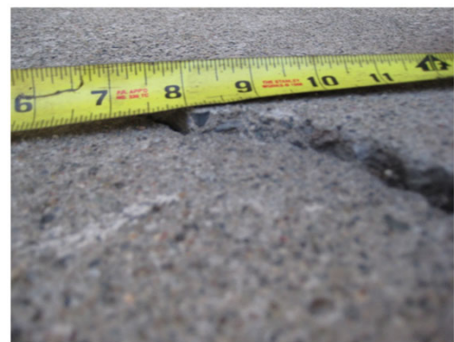
This concrete is cracked and shows vertical offset-should be checked and repaired
