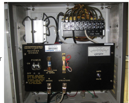
Impressed current system rectifier—this requires periodic readings to determine if system is providing sufficient cathodic protection
