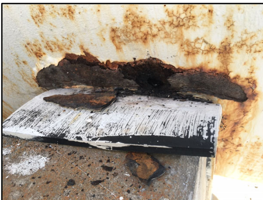
Aggressive corrosion at tank support; black material is wear pad placed between concrete support and tank
