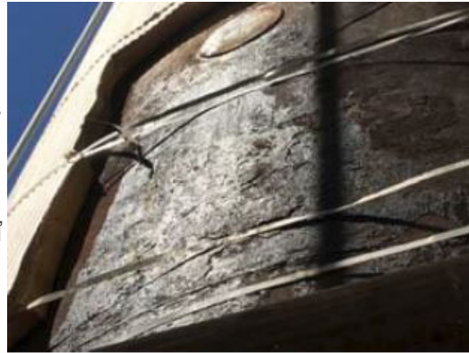
Example of corrosion found beneath insulation
