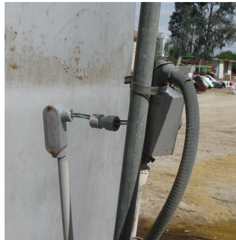
Exposed wiring next to tank storing flammable liquids
