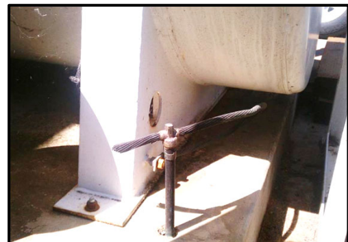
Ground rod and bonding cable installed for a fuel AST
