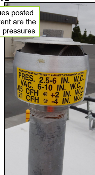
EVR rated pressure vacuum vent on gasoline AST
