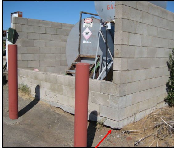
This photo shows some washout of the secondary containment berm of this tank system, but not the tank itself
