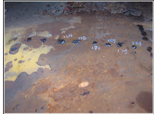
Corrosion on flat surfaces inside emergency generators can occur from rainwater intrusion into the enclosure. The only way to quantify how bad is corrosion is through ultrasonic thickness (UT) testing to determine the remaining steel thickness
