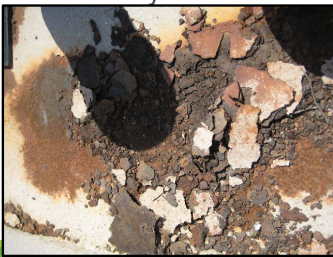
Substantial corrosion found on a tank located in a coastal area
