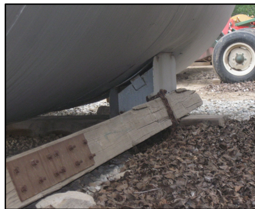
Unconventional or field engineered foundations are clues that UST might be being used as AST
