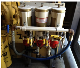
Filter system on emergency generator
