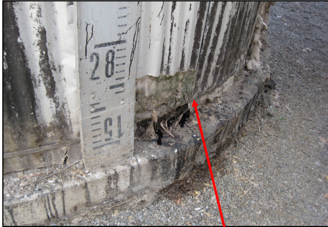
Green colored mold/mildew found on this tank
