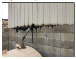
The base on the outer wall of the shed was stained with used oil.
