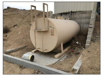
A household hazardous waste (HHW) facility was collecting used oil from the community into a used oil tank. On the inspection, it was noted the tank appeared to be in good condition. The secondary containment consisted of a concrete base and 3 berms approx. 5 inches high. The secondary containment was filled with sediment, dead plant matter, and other types of debris.
