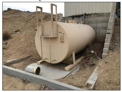
The facility was unable to provide evidence that the 500-gallon used oil tank had undergone a tank assessment. The tank was installed in 1996. On the inspection, it was noted the tank appeared to be in good condition.
