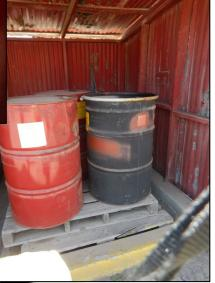
Inspectors observed three (3) 55-gallon drums stored on a wood pallet within a concrete-bermed secondary containment area with illegible hazardous waste labels affixed to each drum. A total of approximately 165 gallons of used oil (California Waste Code 221) was cited in violation.
