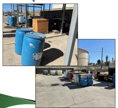
Inspectors observed approximately sixty-five (65) 55-gallon drums stored on wood pallets and twenty (20) 250-gallon plastic totes stored without hazardous waste labels in a concrete-paved storage area. A total of approximately 8,500 gallons of various hazardous wastes including asbestos, used oil, and petroleum-impacted soil were cited in violation.
