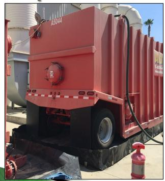
Inspectors observed a treatment tank did not have adequate secondary containment at an LQG. A small plastic liner was placed around the base of the tank, but the liner was not sufficient to contain the volume of the contents in the tank (approximately 21,000 gallons). The tank was "temporary" and single-walled. The contents were paint-related wastes with Chromium (D007).
