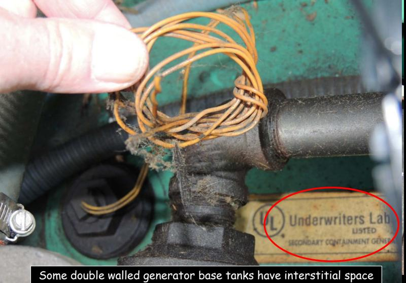
Some double walled generator base tanks have interstitial space leak sensors... and some of those are not connected  $\odot$
