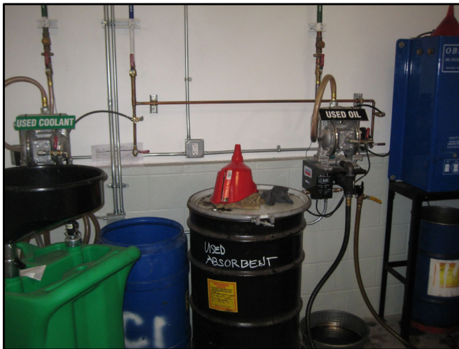
Oil collection station where oil from oil drains and receivers is connected via quick-connect fittings, then pumped by diaphragm pump to tank
