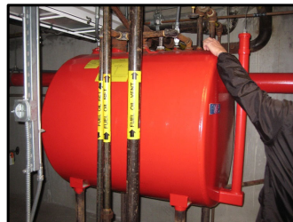
Fire pump tank
