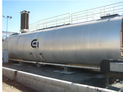
Insulated tank storing asphalt—not in APSA, but included in SPCC
