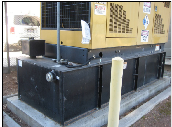
Emergency generator with sub-base tank
