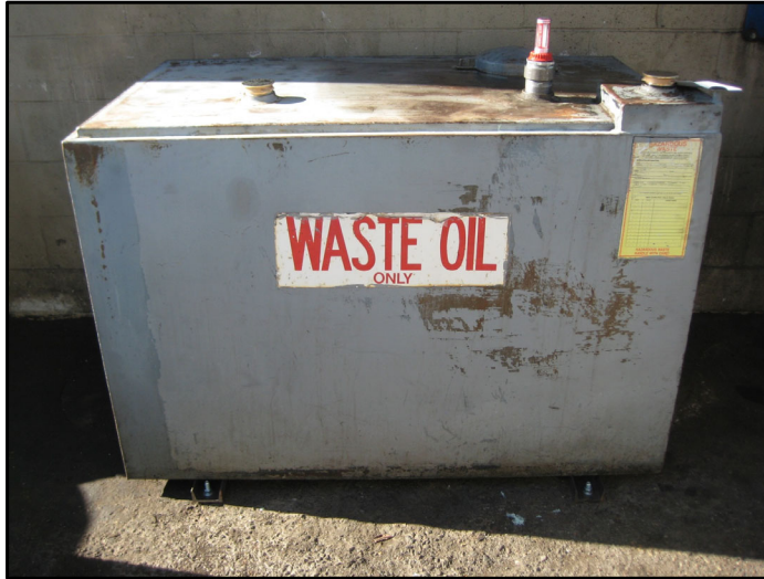
Simple, stand alone 2X walled tank, oil poured by hand to fill
