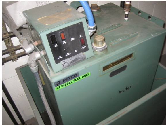
Small day tank used for this emergency generator system
