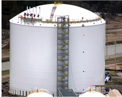
Ammonia Storage Tank built to API 620
