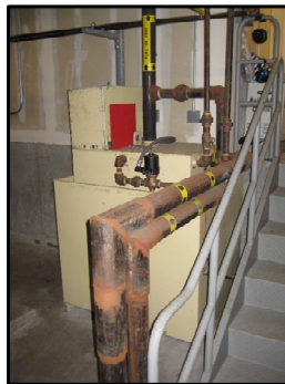
Day tank for emergency generator
