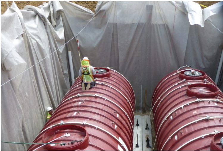
Underground Storage Tank (UST)
