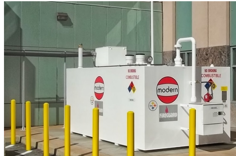
Aboveground Storage Tank (AST)
