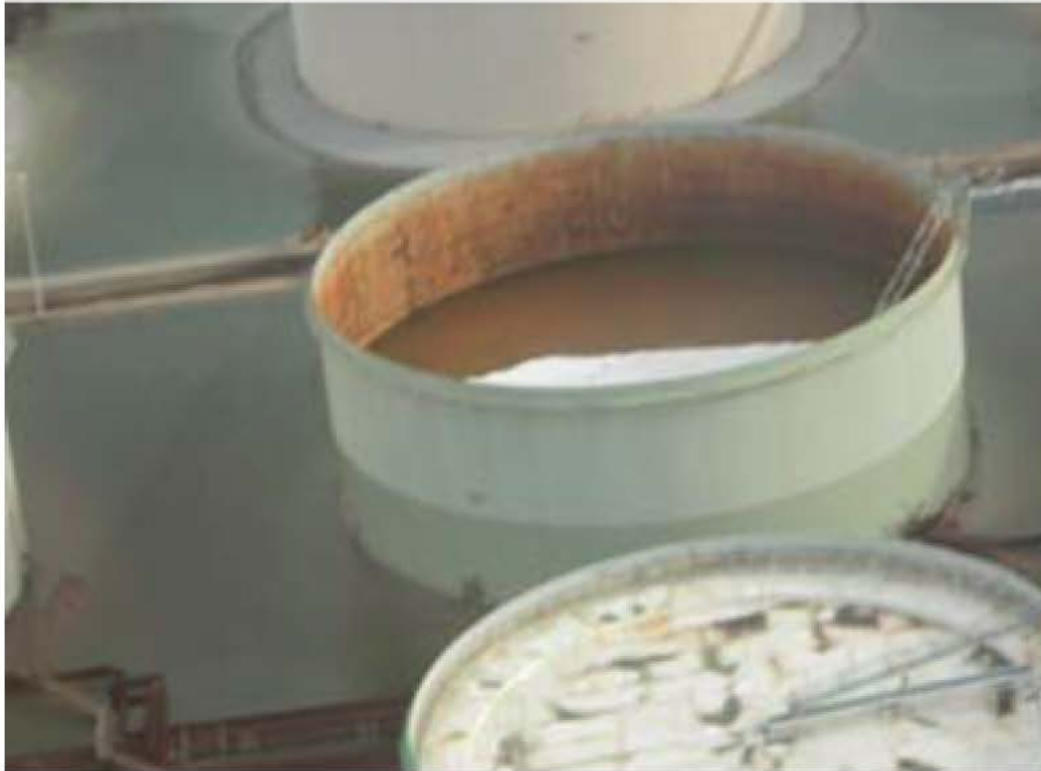
Figure 39 Inadequate precipitation drainage
