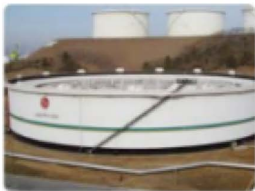
Floating Roof Near Top
