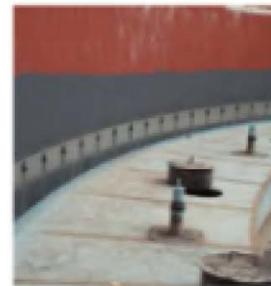
Floating Roof seal
