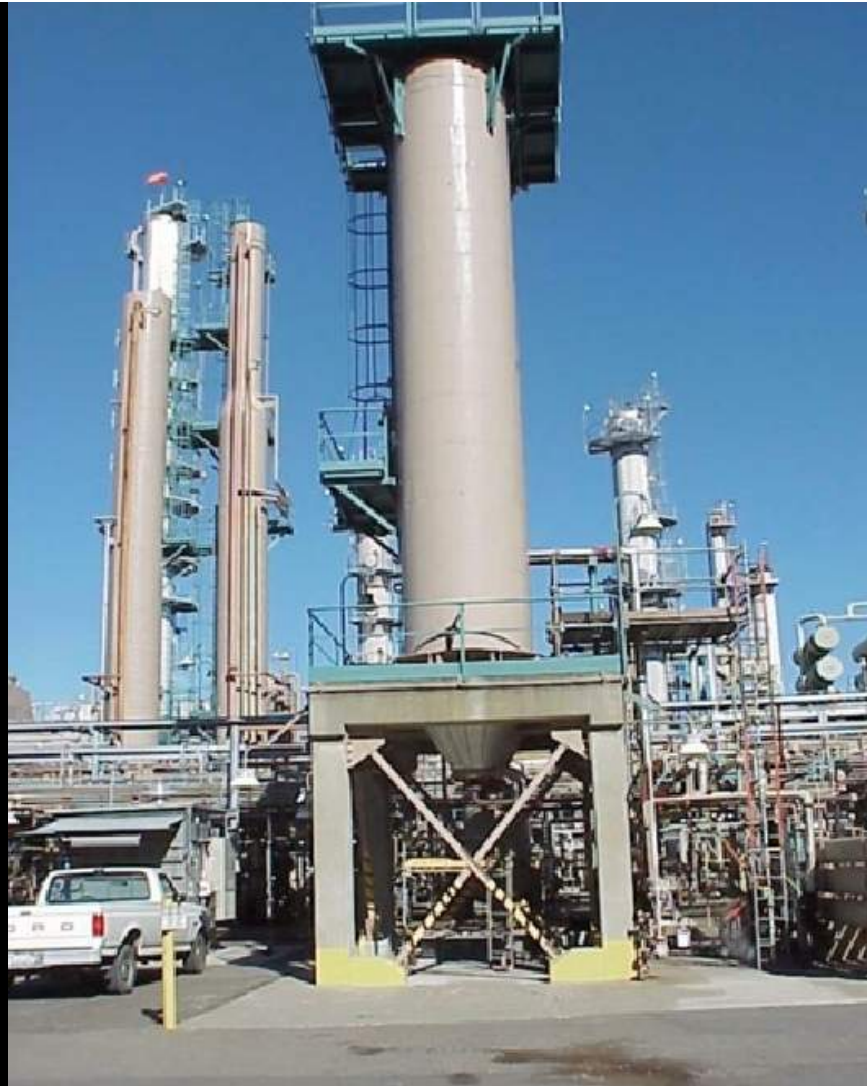
Retrofitted Slender Concrete Table Top
