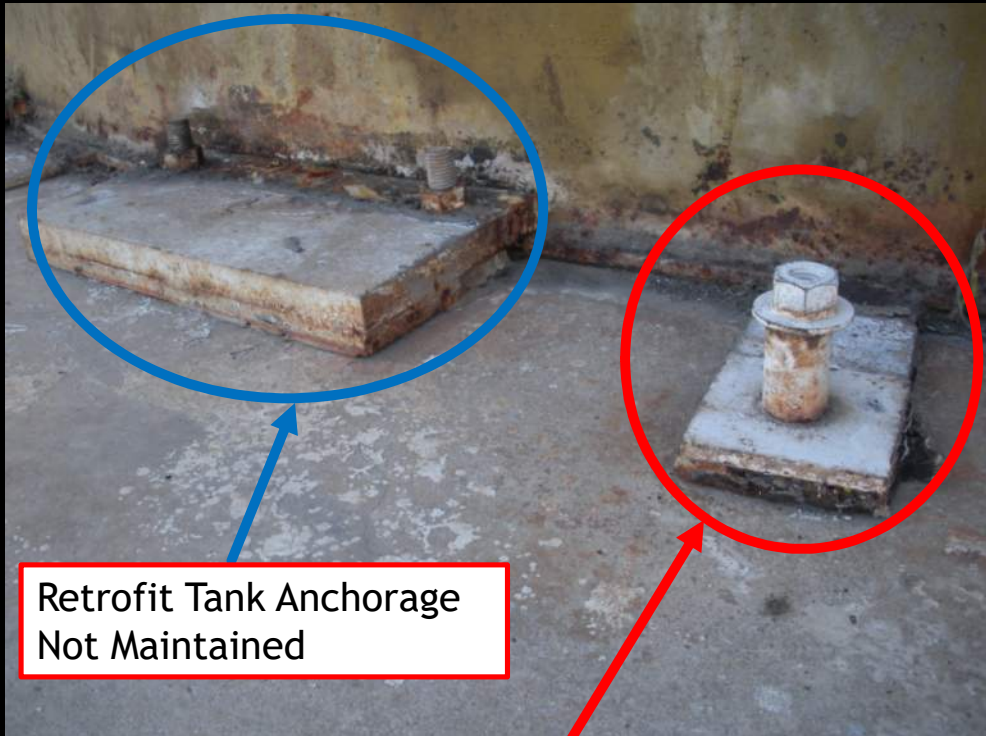
Original Tank Anchorage Highly Suspect
