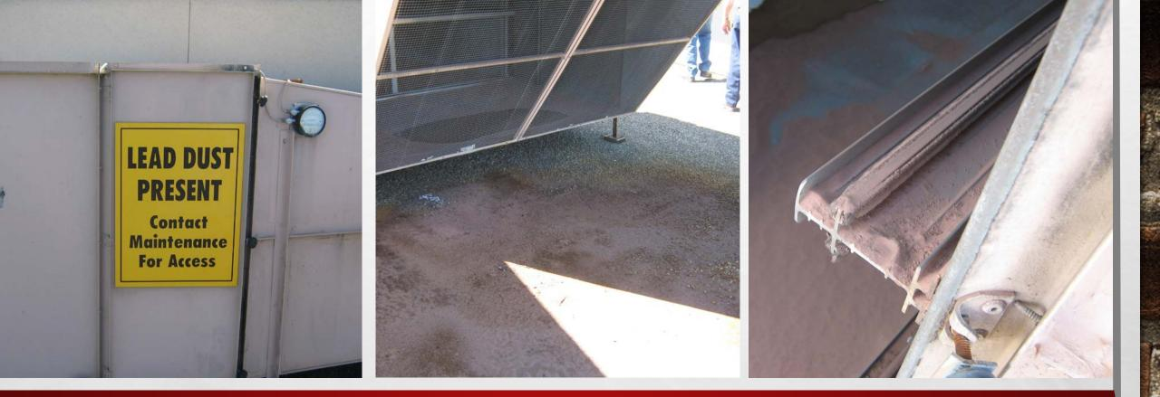
INADEQUATE FILTRATION SYSTEM. COPPER DUST CONTAMINATION THROUGHOUT ROOF AND SURROUNDING AREAS. THIS RANGE WAS SHUTDOWN
