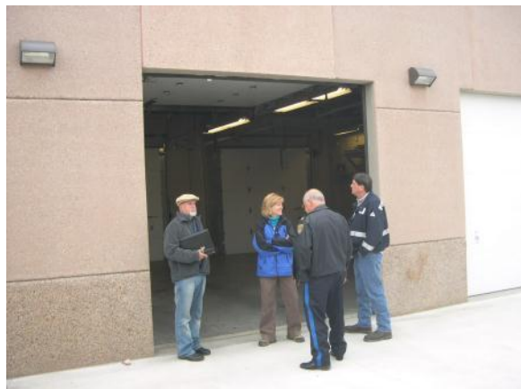
1. Odors reported in new bldg
