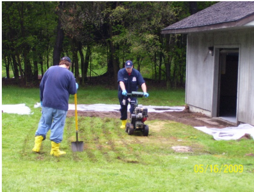
Photograph 9-16 View of a soil/sod cutting operation
