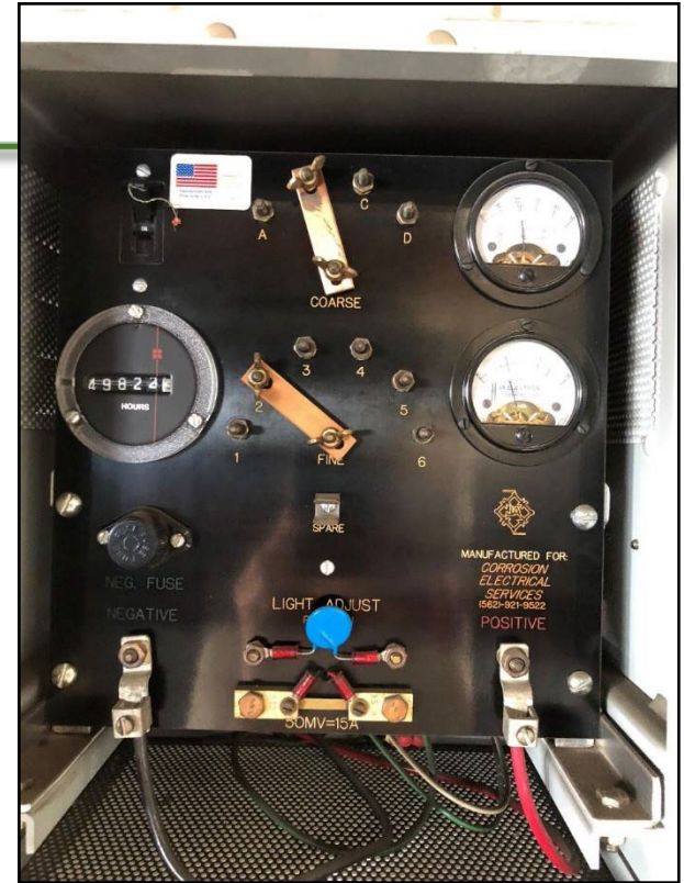
Cathodic protection rectifier panel
