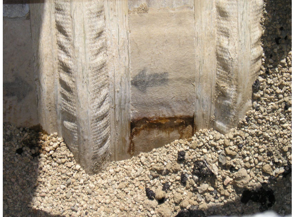
SW Tank with broken seam
